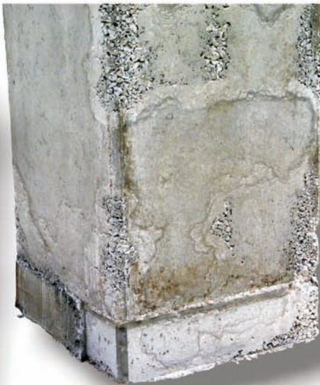
With high-cycle vibration in congested rebar
